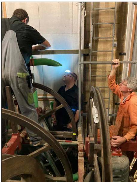
*Looking sideways on at the curved section of ducting above the treble, positioned to catch the two o'clock strike*
